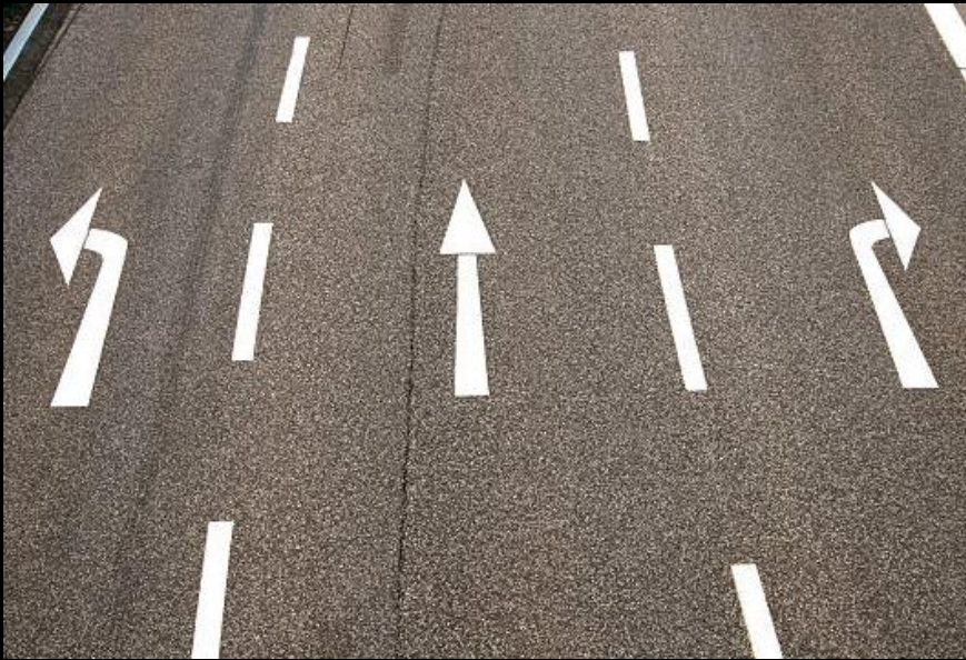
Transverse markings (e.g., arrow markings)
