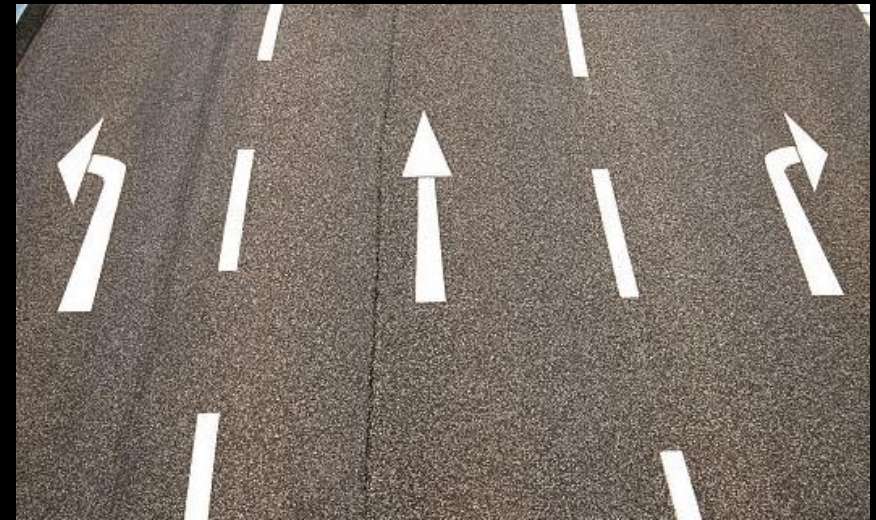
Transverse markings (e.g., arrow markings)
