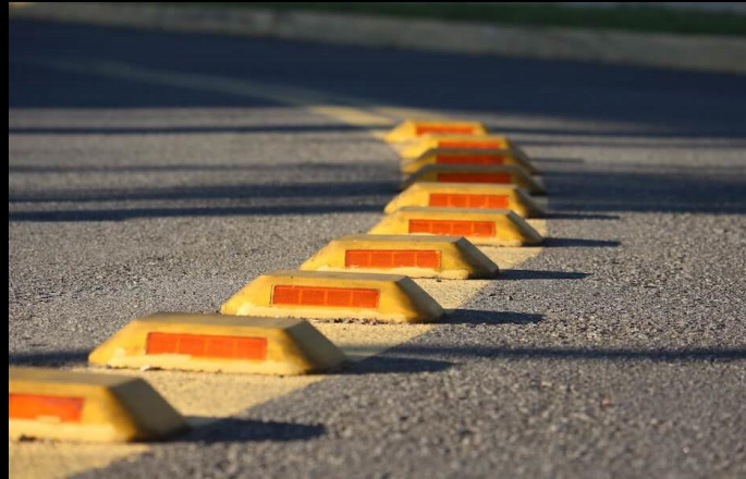
Raised pavement marker
